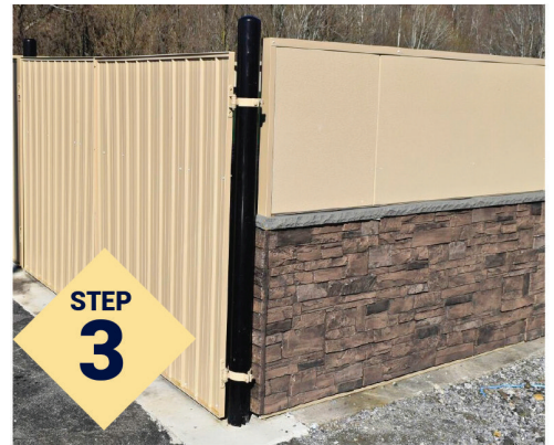
Install the Urestone brick or stone paneling onto the siding surface and install the gates.
